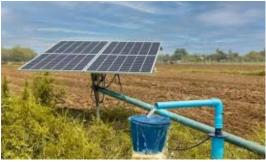
Fig: Photovoltaic Water Pumping
