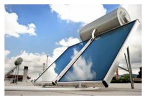
Fig 2: Solar Flat Plate Collector
